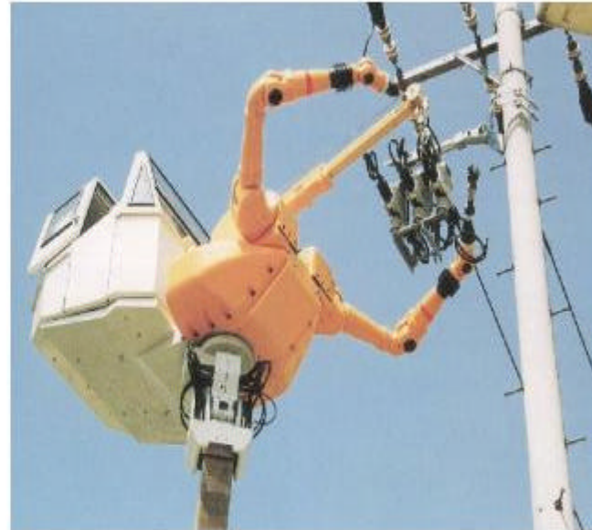
High Power Line Maintenance Robots (Kyushu Electric Power/Yaskawa)
